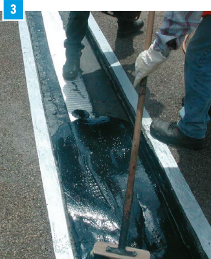
Applying the hot Nafutekt Plus to joint
