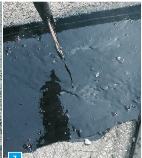
Pouring hot Nafutekt Plus onto and into aggregate
