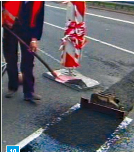
Application of coated 1 – 3 mm chippings, followed by sweeping-off of excess
