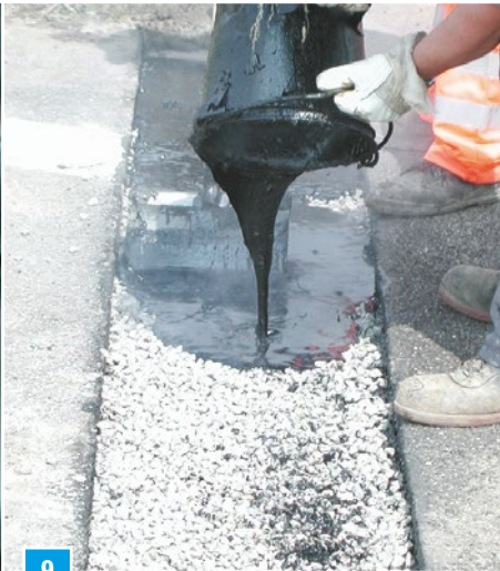
Pouring the final layer of Nafutekt Plus
