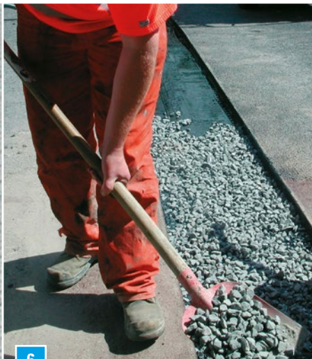
Placing and compacting heated aggregate in 3 cm layers
