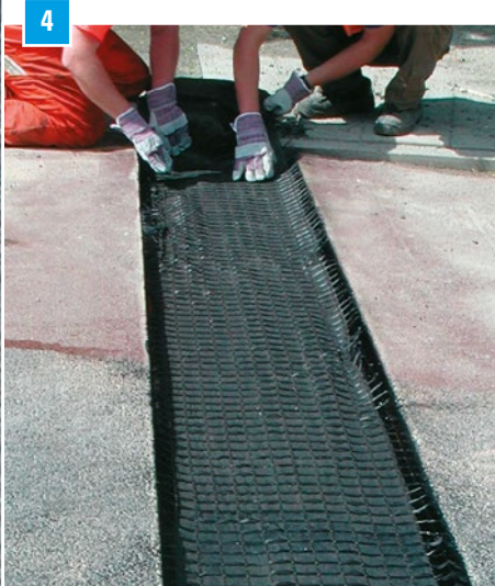
Laying the pre-cut, heavy-duty polyester mesh
