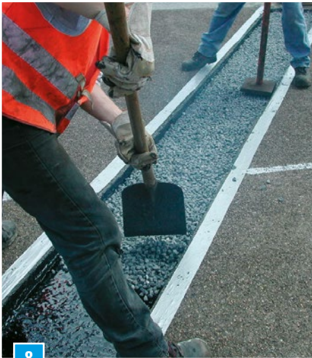
Placing and compacting a second 3 cm layer of aggregate
