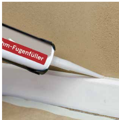
Filling a joint along a skirting board using natural white filler
